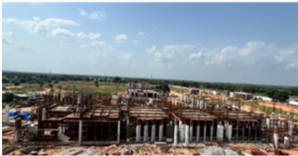
Ground Floor Roof Slab Works under progress
