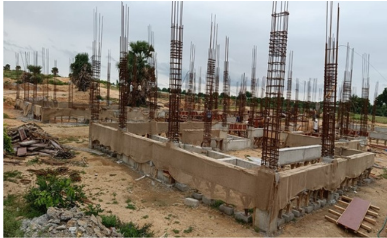
Plinth Beam works under progress
